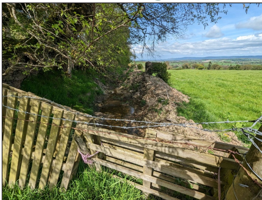
This is a bridleway in the middle of the countryside SW of Denbigh. Apart from the obvious barrier the surface has been dug up. SH999632 (photo: Tom Marshall)
