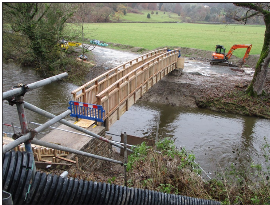
The new bridge should soon be ready for public use.
